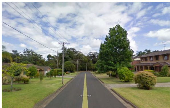
Figure 16 Ulandi Place adjacent one and two storey dwellings close to road frontage
